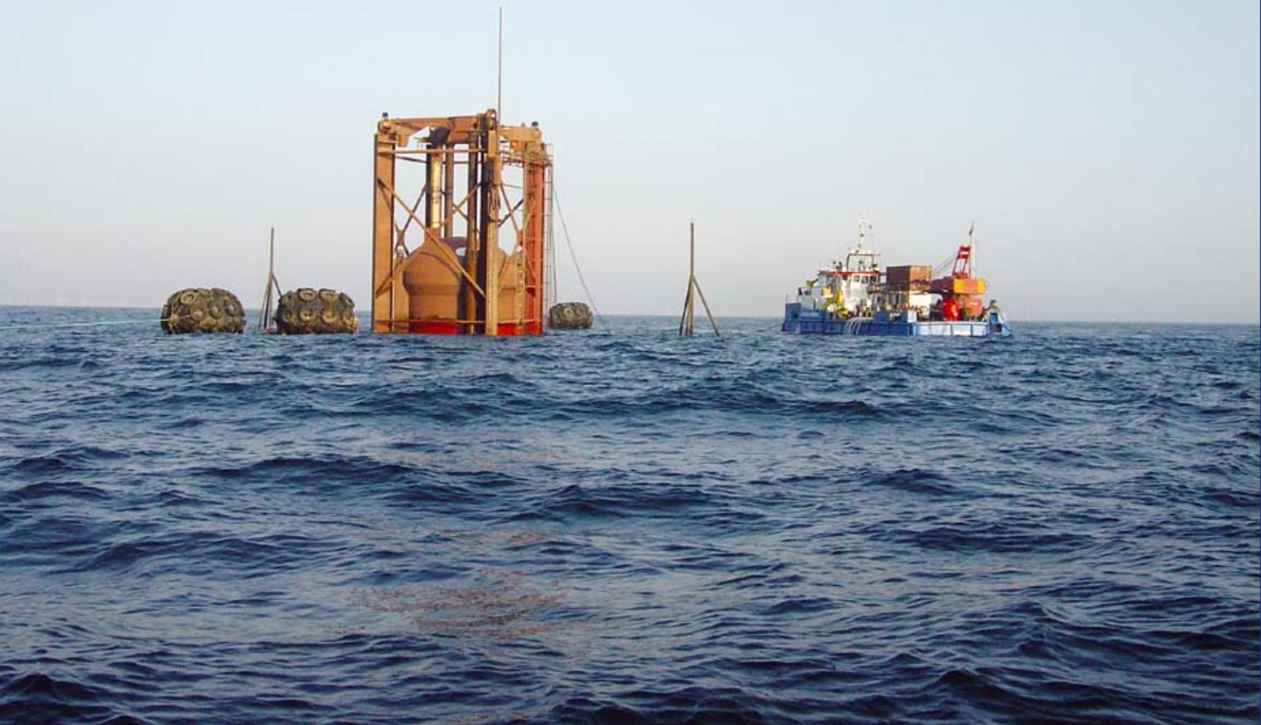
The Archimedes Wave Swing, a wave energy converter, being submerged in the Atlantic ocean off the northern Portuguese shore on 19 May 2004.
