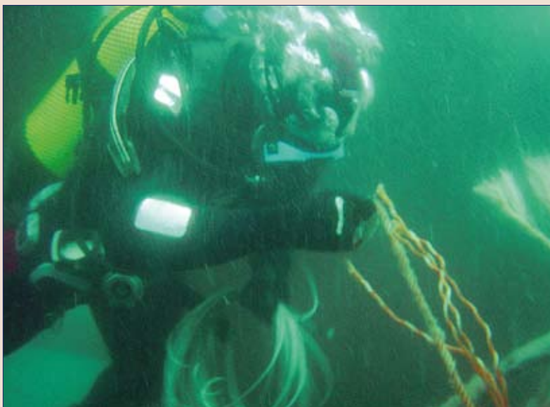
Since the electric shore controls for the valves and pumps did not work, divers established a link that would enable them to be operated from on board the ship.
