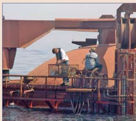
12.45 p.m. Ir. Michel Damen and Jan-Willem Vroege fix a last-minute connection with a level sensor that will measure the level of the water in the central compartment.
