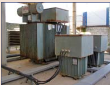
The 3000 volts coming from the thyristors is fed to a transformer to step up the voltage to 15 kV.
