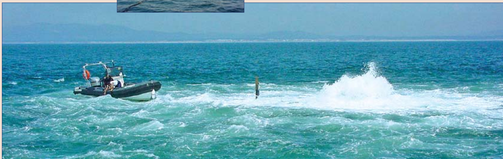
19 May 2004, 5.00 p.m. A diver having opened a valve, water flows into the AWS interior, forcing out the air to add weight to the pontoon in order to obtain the correct air spring characteristics.
